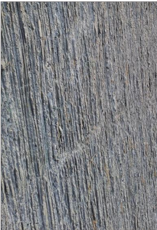
Figura 26 – Texture casseforme in arelle
